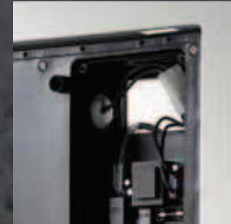
Soft Start device to reduce motor consumption during start up
